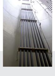
Towerbuss for Down-Tower Power Transmission
